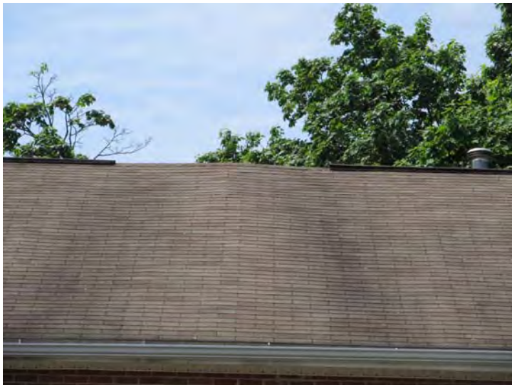
Original roof shingles exhibit age-related wear
