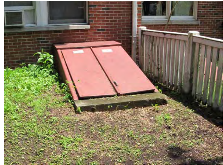
Each unit has a steel bulkhead door for basement access – No significant rust or damage noted
