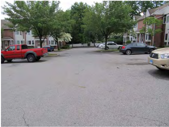
Typical original asphalt paving – No significant wear or damage noted
