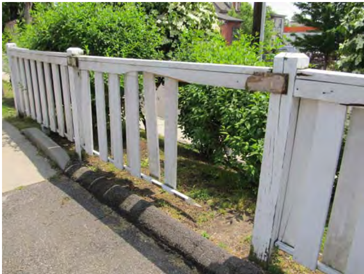
Original wood fencing is in poor overall condition – Replacement scheduled for completion in 2013
