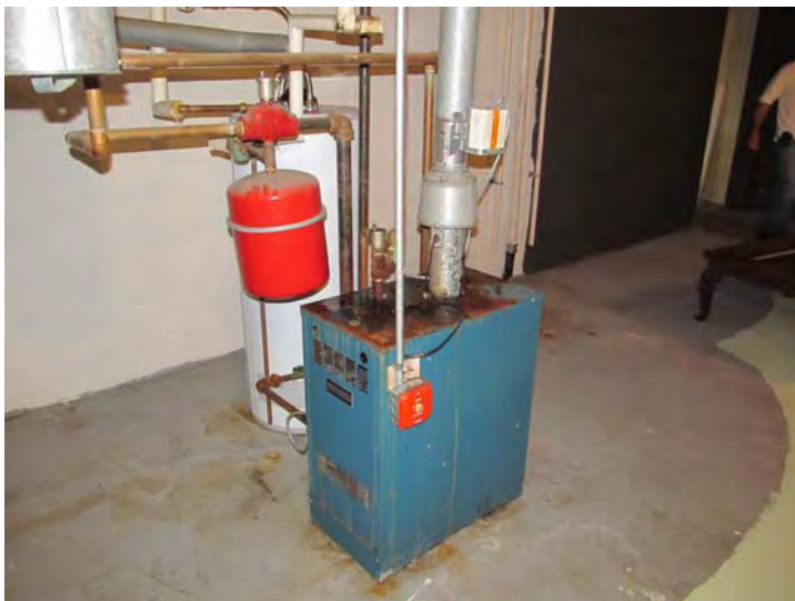
Typical natural gas-fired boiler and domestic hot water tank found at the basement level of each unit
