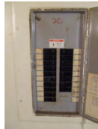
All units have electrical load centers equipped with circuit breakers
