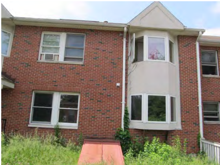
Brick veneer and EIFS exterior wall surfaces are in fair condition
